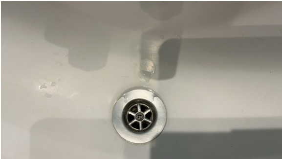
Riss i vask
