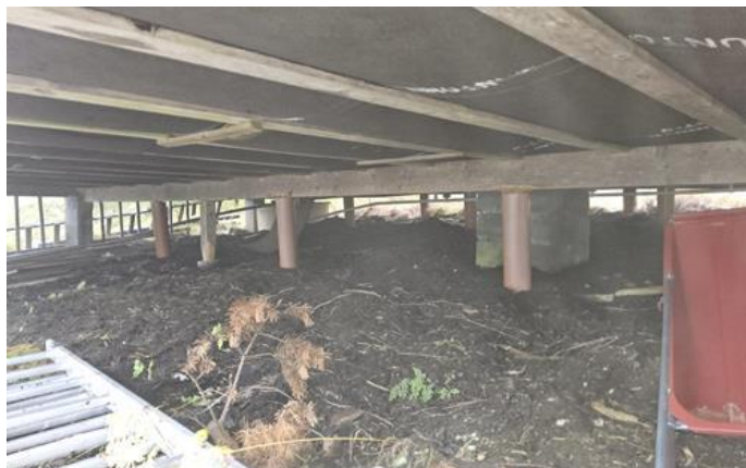
Grunnmur, fundamenter - [IMG_20241017_104240]
